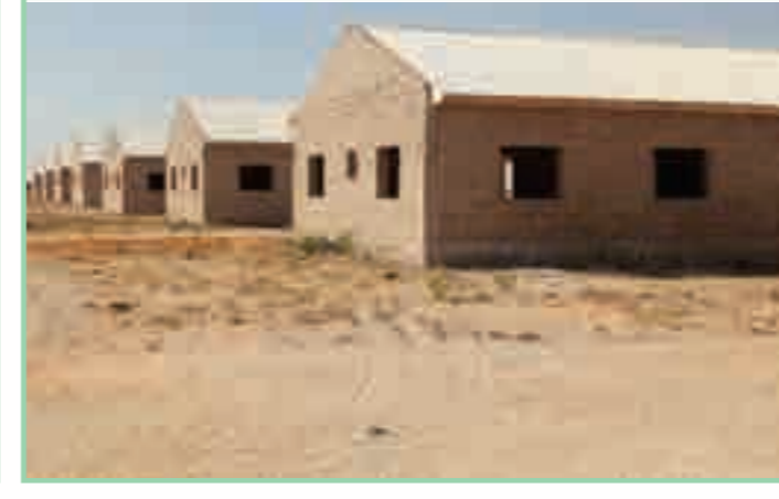
1800 housing units under construction across the state.
