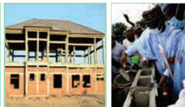
Damaturu Modern Market under construction
