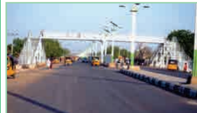
Damaturu overhead bridge
