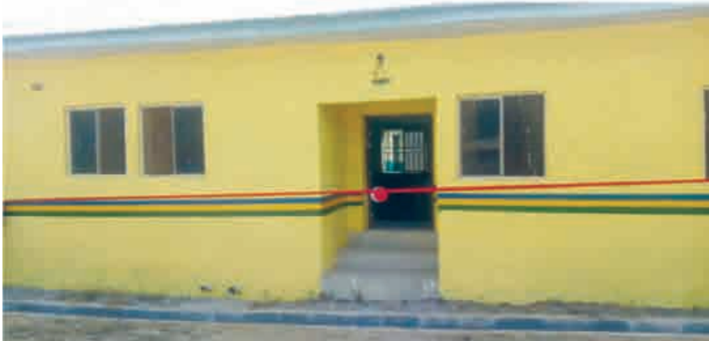
■ The police station built and donated by the Ogidi community
