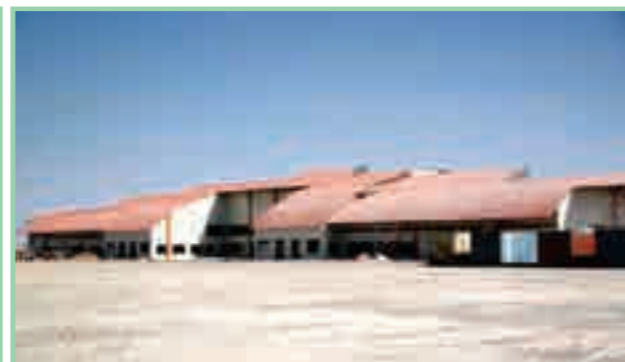
Cargo Airport Building 1
