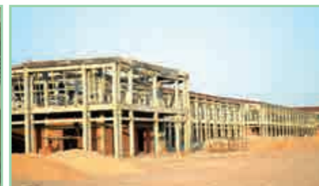
Damaturu Modern Market under construction
