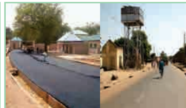
Township road under construction Buni Yadi 1
