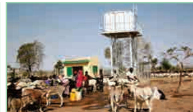
Rural Water supply
