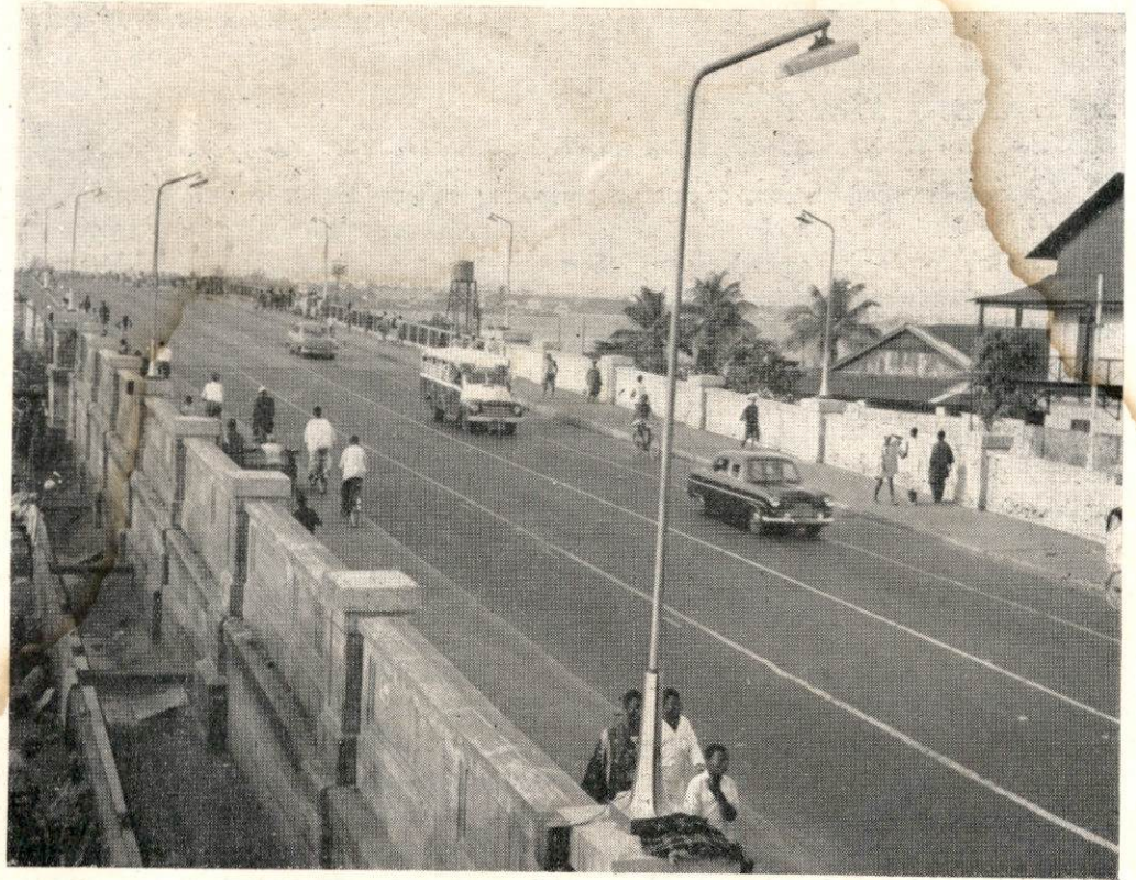
Carter Bridge seen from the Lagos end
