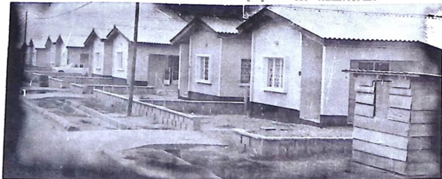
A section of Government's Housing Estate.
