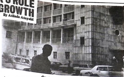
Central Bank building.
