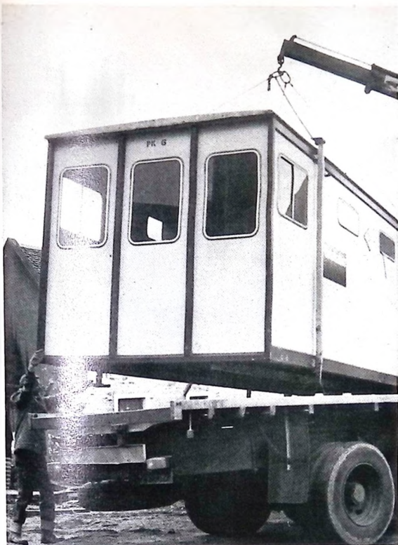
Portacabin is a good example of the relocatable type of system.
