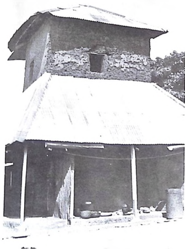
ODOGO, the oldest building in the Palace grounds is thought to originate in 16th century. It was used as a lookout for enemies or traders on the river Niger and for the procurement of customs duties from northern merchants, trying to reach S. Nigeria and the sea.
