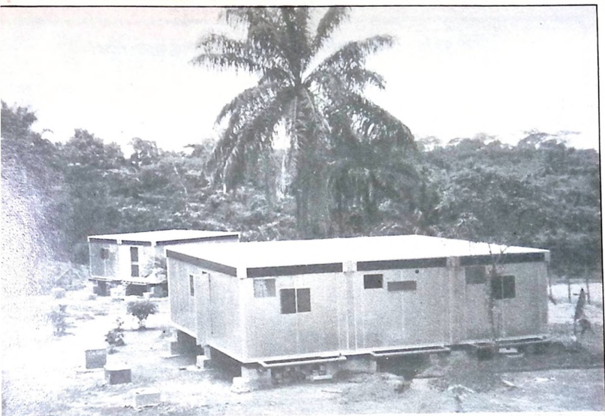
Accommodation for staff of Ove Arup & Partners, Monrovia using Terrapin's high duty export units, delivered in knockdown form.
