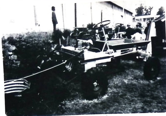
A Tinkabi on show powering an irrigation pump.
