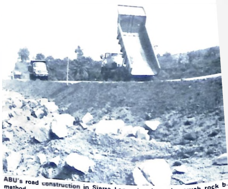
ABU's road construction in Sierra Leone involves the crush rock method.
