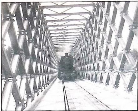
Modern bridge design. The Mann/Krupp D Bridge MS317/3 which is single storey, double truss with 3rd chord, double lane with roadway hollow multistrut steel plates.
