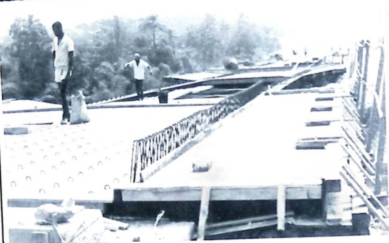
Part of ABU's bridge construction programme in Sierra Leone
