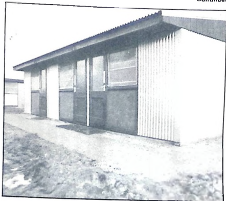
A Hallam Panelpac bachelor dormitory accommodation factory clad with aluminium alloy.
