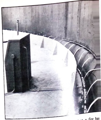
An alternative extinguishant for roof tanks using BCF.
