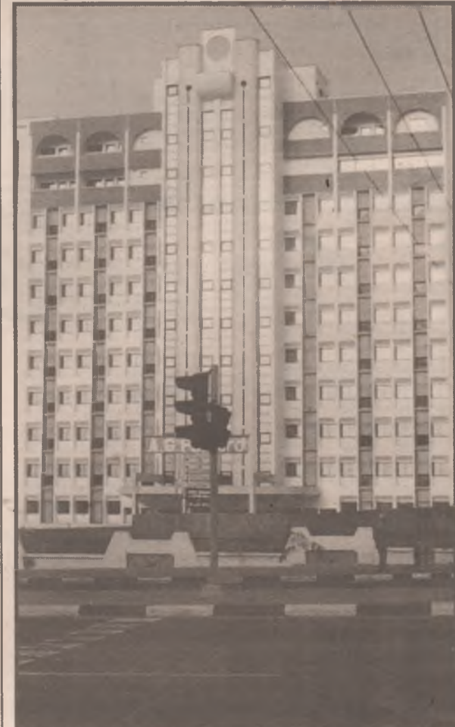
The magnificent Bank of the North Headquarters at the Central Business District, Garki, Abuja, just completed.
