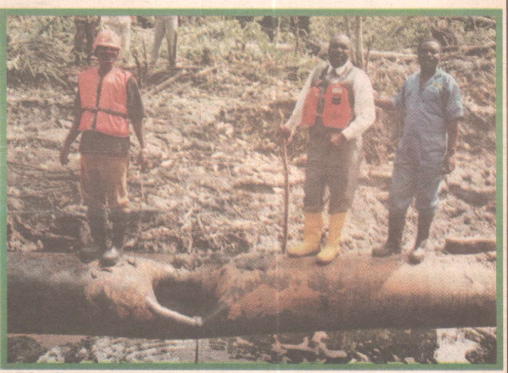
NNPC engineers on top of the damaged pipeline.
