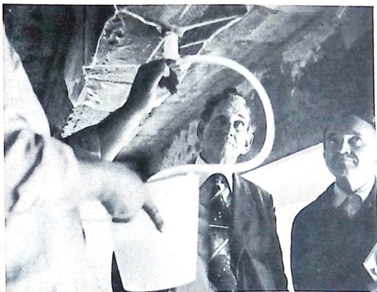
Repairing faulty reinforced concrete beam by vacuum impregnation, Italy.
