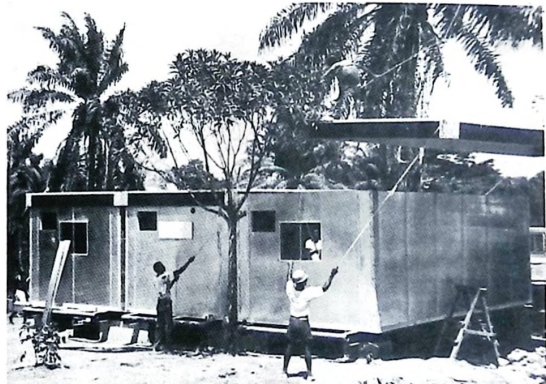
Easy and quick erection is an attractive aspect of systems building.
