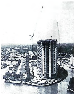
Lorain MCB150 tower crane.
