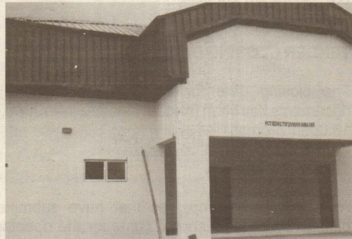
THE repaired building at Government Science Technical College, Area 3, Garki, Abuja.
