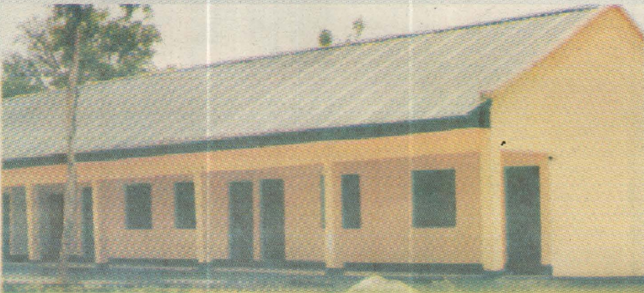
One of the modern classroom blocks constructed by the Doma administration.
