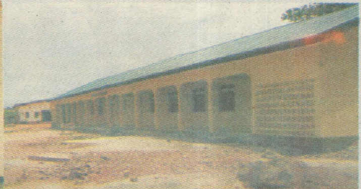
Newly Constructed Biology Lab. at College of Education Akwanga
