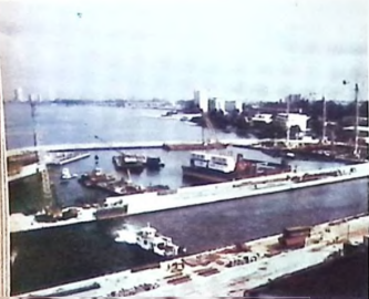
Construction of Naval Dockyard, by Spibat Nigeria Ltd
