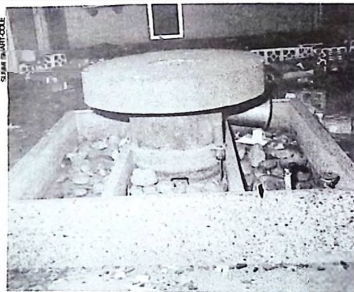
• The water fountain in Alhaji's house. It was destroyed during the riot
