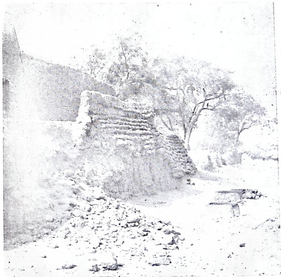
The City Wall of Wurno: north west now delapidated
