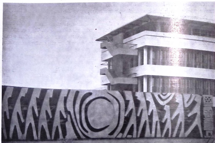
Sculptured Mural, 'The Art of Understanding' by Erhabor Emokpae of tooled concrete which exposes the granite aggregate standing in front of a wall faced with mosaic of predominantly blue colour. The main four-storey block is behind
