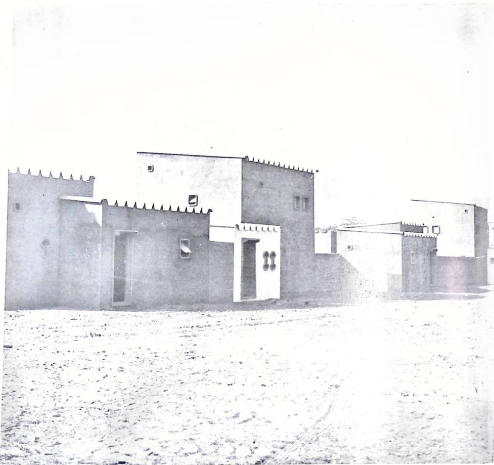
Part of the township of Yekca, the head of navigation on the future lake, which has been rebuilt. The houses along the lake shore have been demolished to create space for a quay
