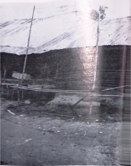
View of tin roof and bamboo walls
