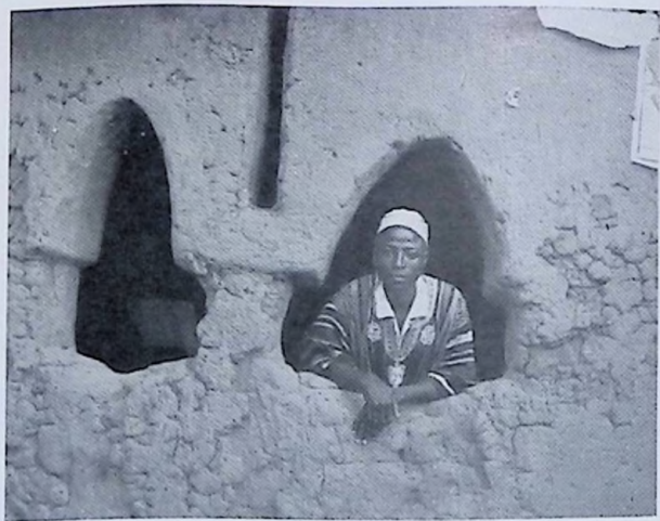
A Window in a Gwari mud hut
