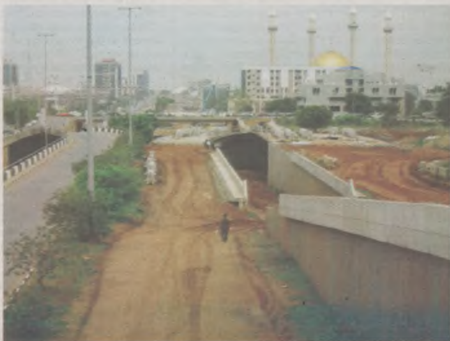
EXPRESSWAY construction within the Central Area of Abuja
