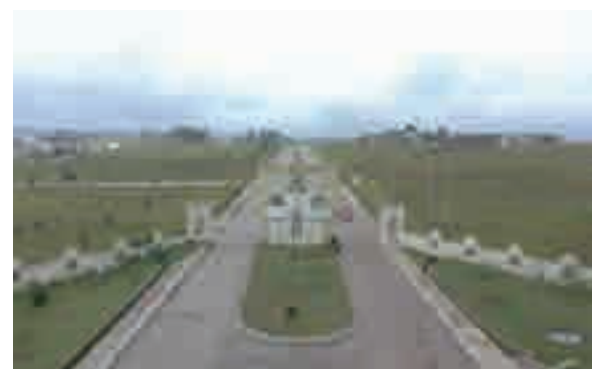
Road network and other infrastructure at the Plateau State University Bokkos 2
