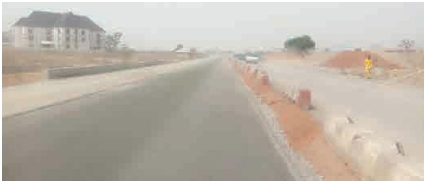
■ Asphalt overlay on the Dutsen Alhaji-Bwari Road is progressing fast
