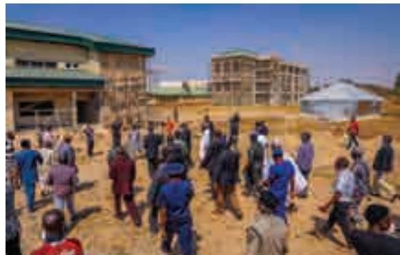
Projects under construction at the Plateau State University Bokkos
