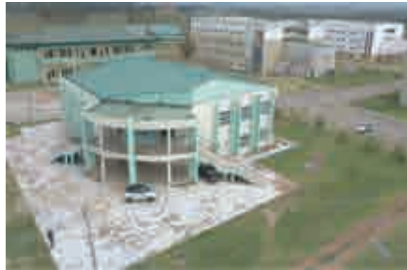
Completed infrastructure executed by Governor Simon Lalong at Plateau State University Bokkos
