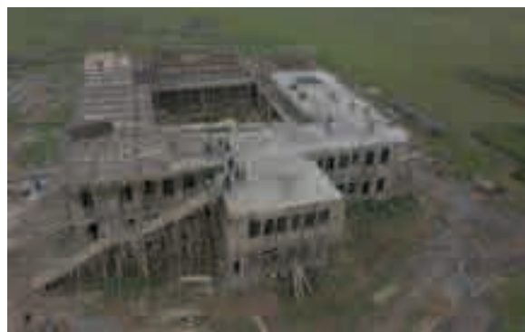
One of the new Faculties under construction at PLASU Bokkos
