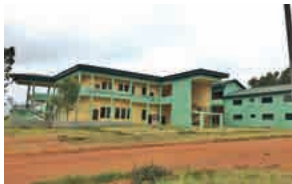
One of the completed structures at PLASU Bokkos
