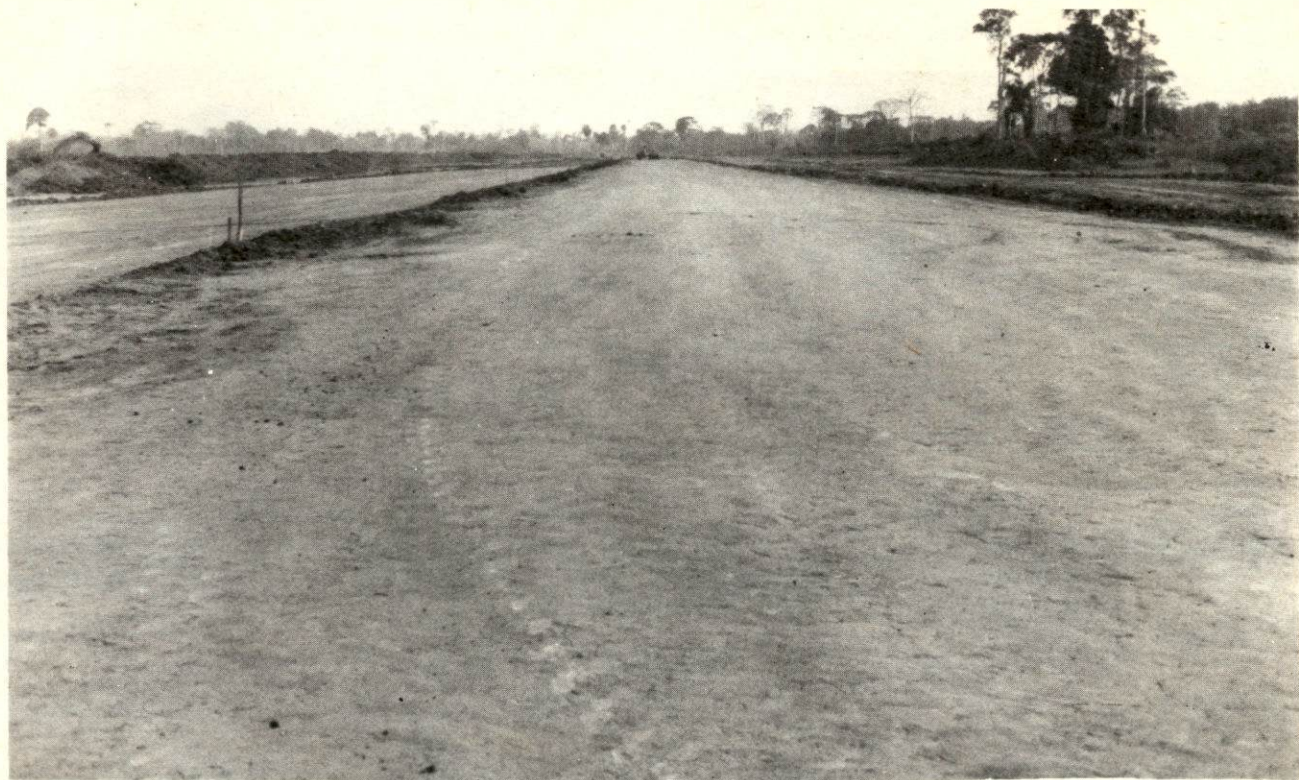
Earthworks of the new Port Harcourt Airport in progress
