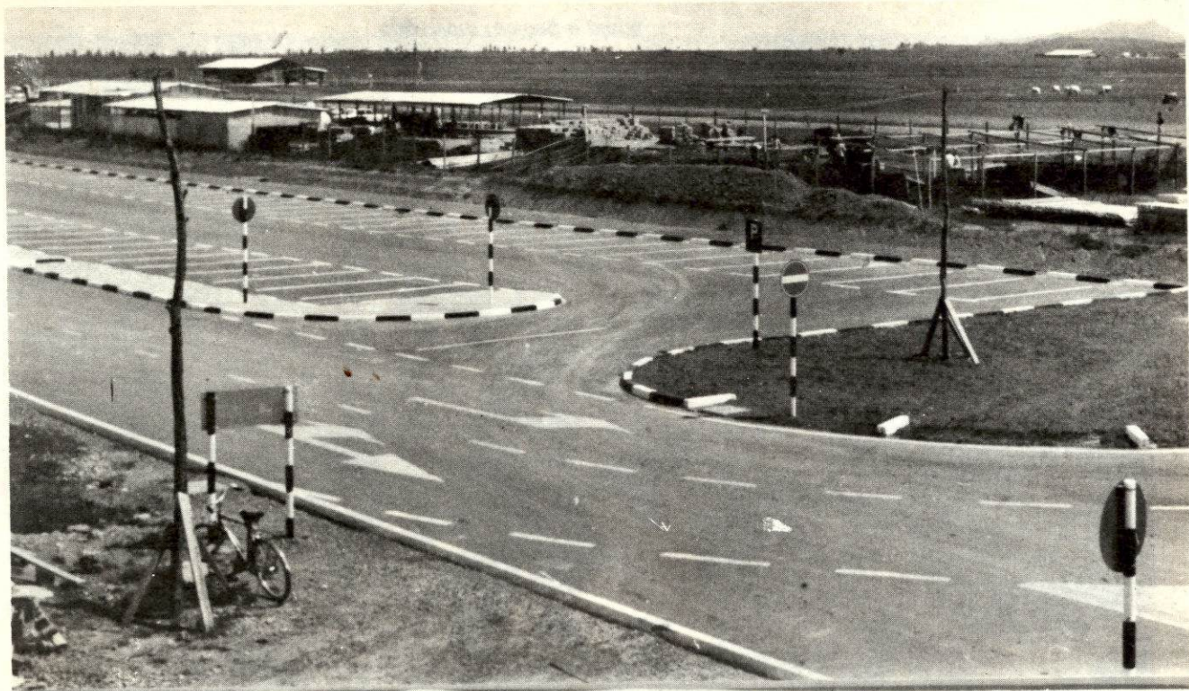
New Jos airport in progress — parking place in Terminal Area
