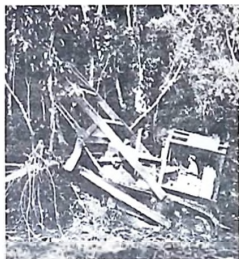
In Ivory Coast the World Bank is supporting the $110m. SODEPALM project, for new palm plantations and attached processing mills. This, the major Ivory Coast agricultural development project, involves clearance of about 70,000 hectares; contract for half of this operation (illustrated here) has gone to JOLKACI, a German contracting firm, which is carrying out the task with about three dozen Allis-Chalmers crawler tractors and a crew of about 250. The European Development Fund of the EEC is the main source of outside finance for this project.
