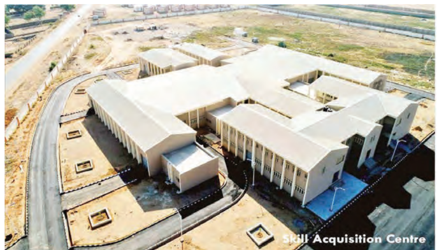
■ Aerial view of the Aliko Dangote Skills Acquisition Centre, Kano that was commissioned by President Muhammadu Buhari on Monday
