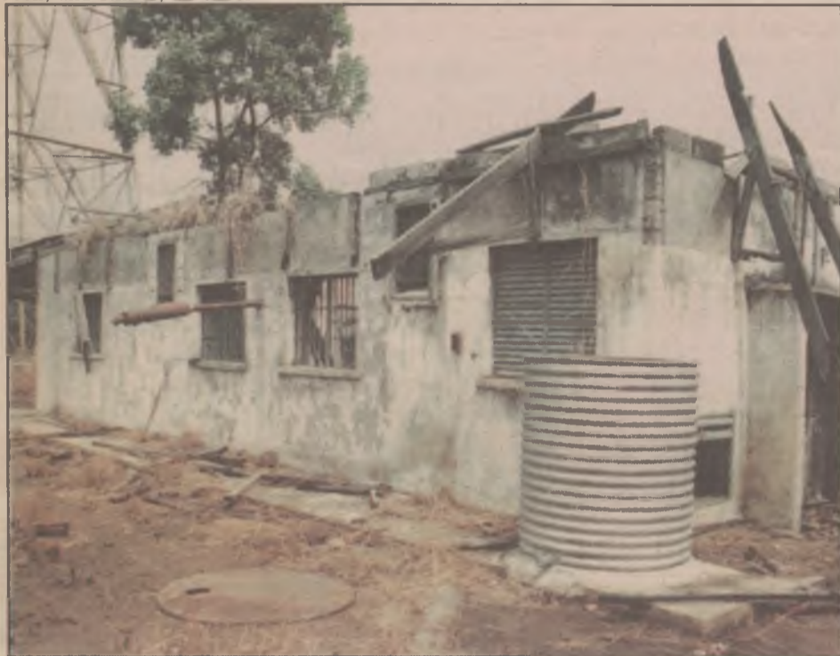
An abandoned building on the hill top
