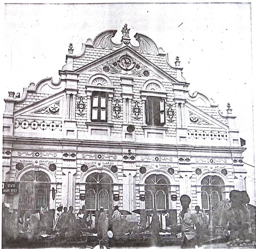
The Old Central mosque with its elaborate façade was built circa 1880. It has been demolished to give way to a new one.
