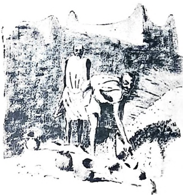
DOMESTIC "SLAVES" REPAIRING A WALL AT KANO.
