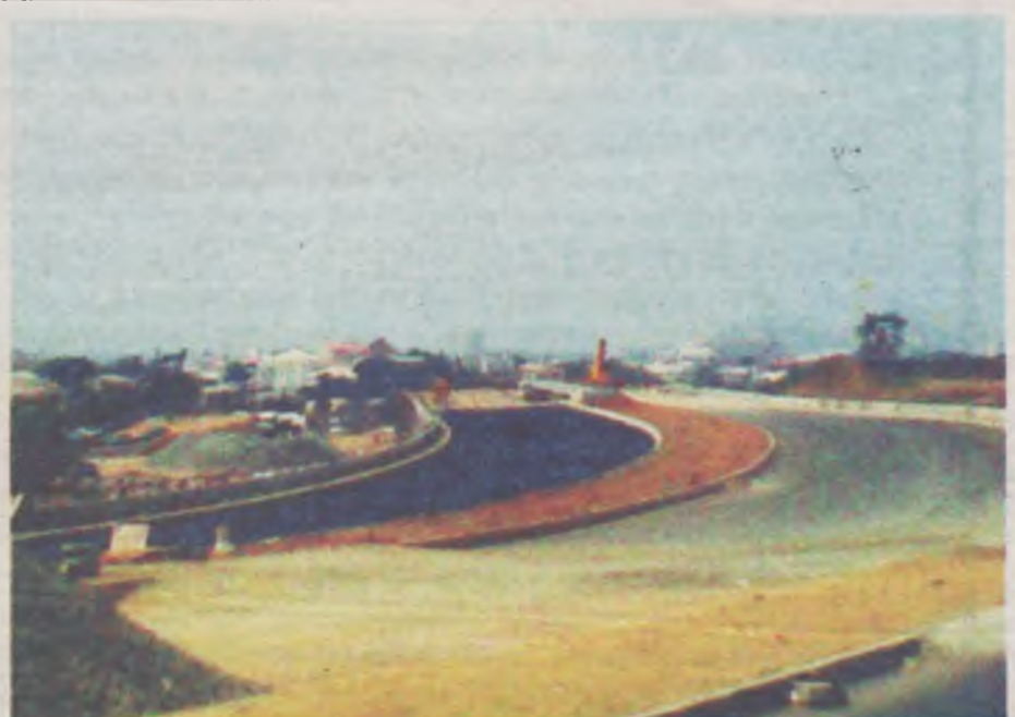
ONGOING construction work at the AYA junction, Abuja
