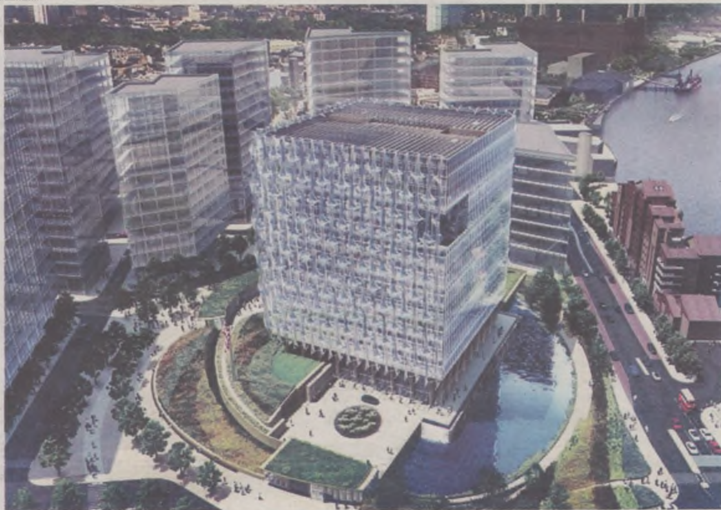
THE new 12 storey U.S. Embassy Thames, London located on the southern bank of the
