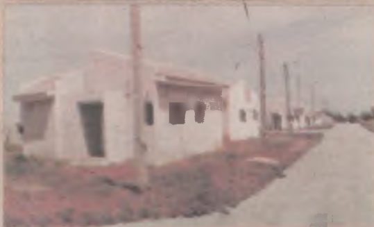
The completed two bedrooms MANA housing estate under the 2,500 mass housing policy
