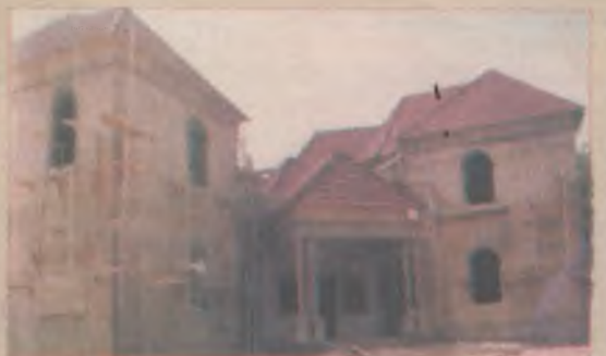
Un-going Government Lodges under construction by the State Government, nearing completion.
