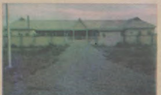
The newly constructed Primary Health Care Centre (PHC) at Wamakko town in Sokoto State all an efforts of providing Health Care Services to the Rural Areas.
