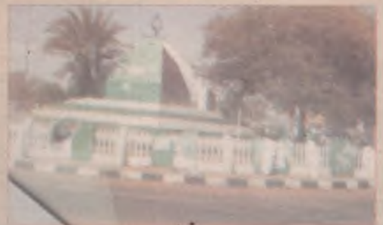
Sokoto Kano road roundabout under going maintenance under the beautification policy of the Sokoto State Government.
