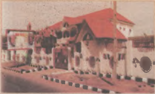
The renovated PDP State Head Quarter Sokoto in preparation for the 2011/2012 Presidential and State Elections. Pix by Triple Cee Media
