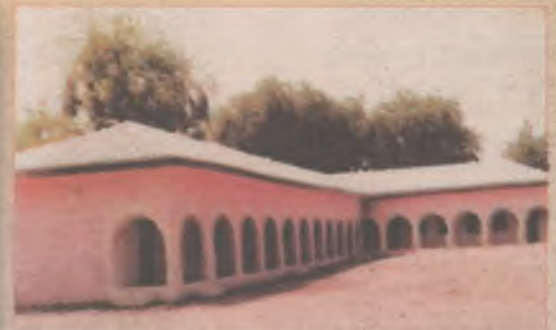
The renovated Turaki House at the old Nagarta College Sokoto, establish in 1905 by the colonial Masters
