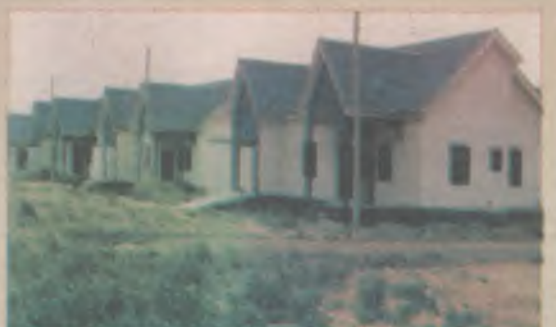
The Bado Housing Project Under the Wamakko 2,500 Mass Housing Policy in Sokoto.
