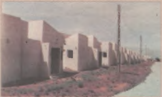
Two Bedrooms MANA Housing Project which is part of the 2,500 Mass Housing Programme by the Aliyu Magatakarda Administration.
