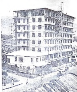
Sierra Leone Electricity Corporation's new headquarters under construction in Freetown.
