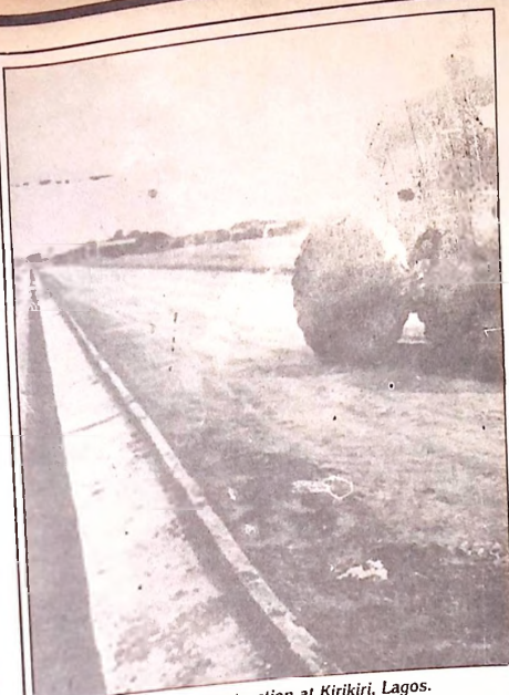
Roads and drainage construction at Kirikiri, Lagos.
