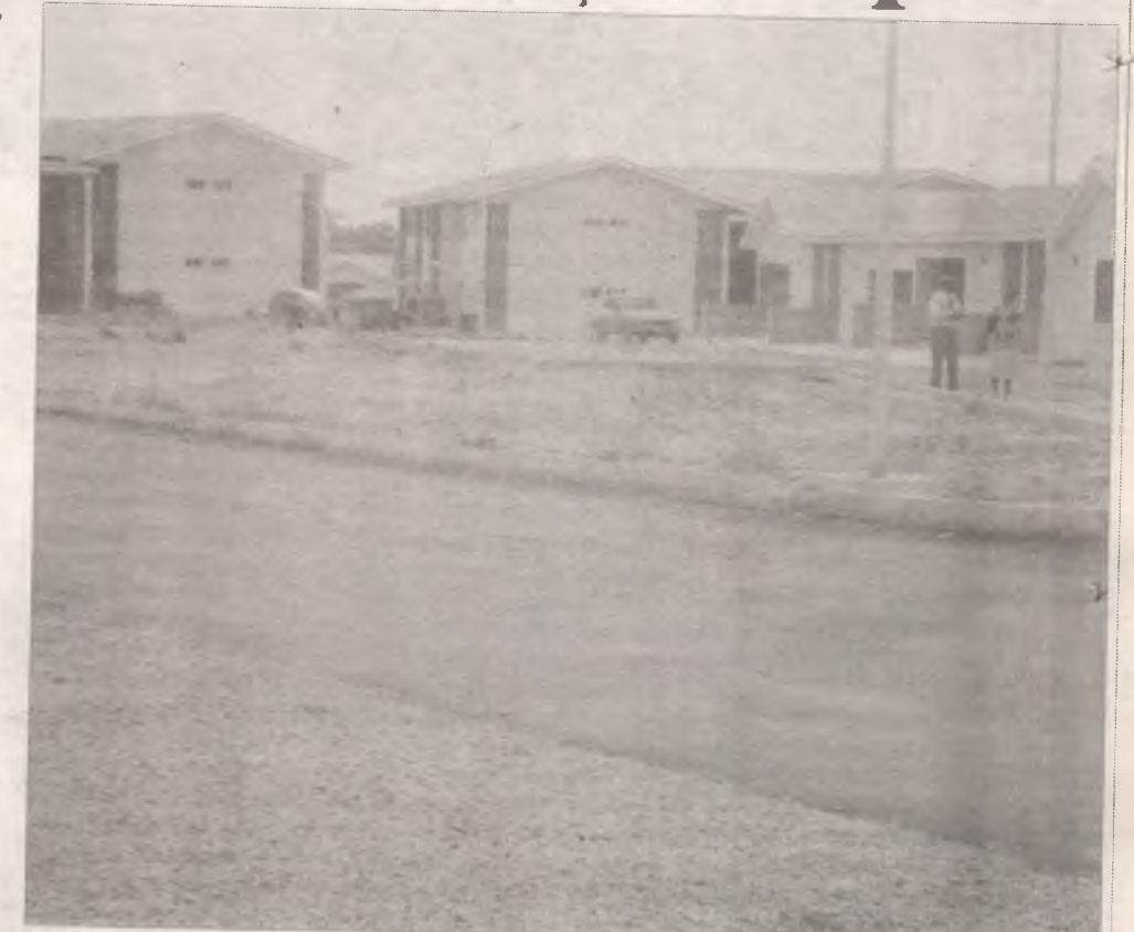
2 bedroom flats financed with National Housing Fund (NHF) but built by Aso Savings and Loans Ltd in Lugbe, Airport road, FCT.
