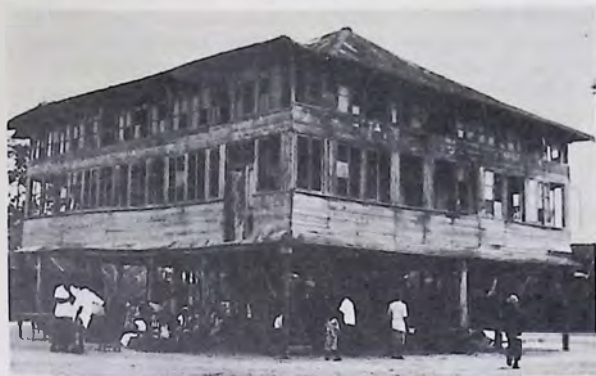
Fig. 80. King Jaja's Palace at Opobo. This wooden prefabricated house, imported from England, reminds us of the short-lived greatness of Opobo.
