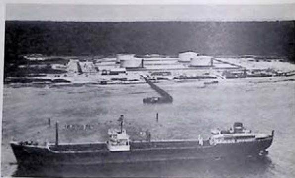
Fig. 57. The oil terminal at Bonny, with an oil-tanker lying offshore in the Bonny River. In the distance the open sea is visible.
