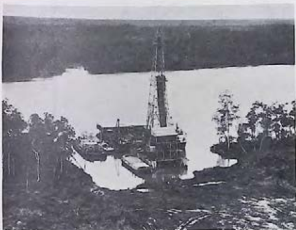
Fig. 58. Drilling for oil in the mangrove swamp forest of the Niger Delta. This well reached a depth of over 14,000 feet before being abandoned.
