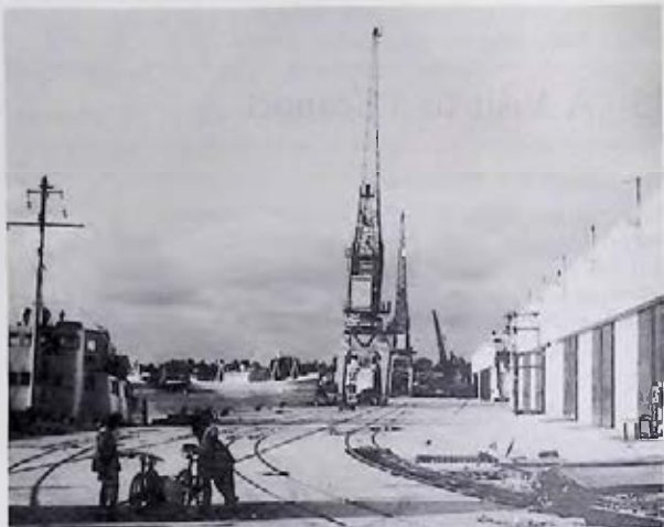
Fig. 63. This photograph shows the newer part of the wharf at Port Harcourt. Notice the rails embedded in the concrete along which the travelling cranes, seen in the background, can move. To the right are the transit warehouses for goods awaiting loading, or awaiting transport away from the wharf. To the left is a smaller motor vessel, in the background three general cargo ships.
