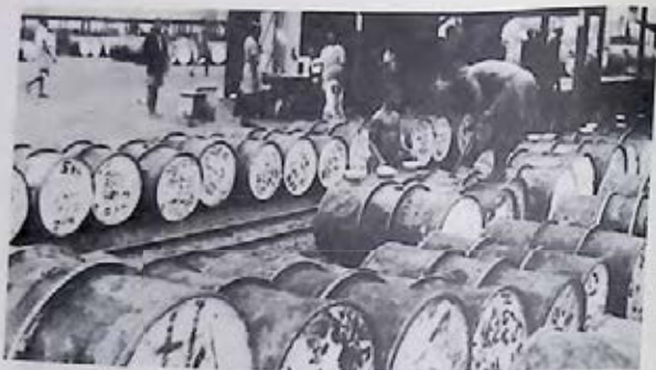
Fig. 34. At the Port Harcourt Bulk Oil Installation.
