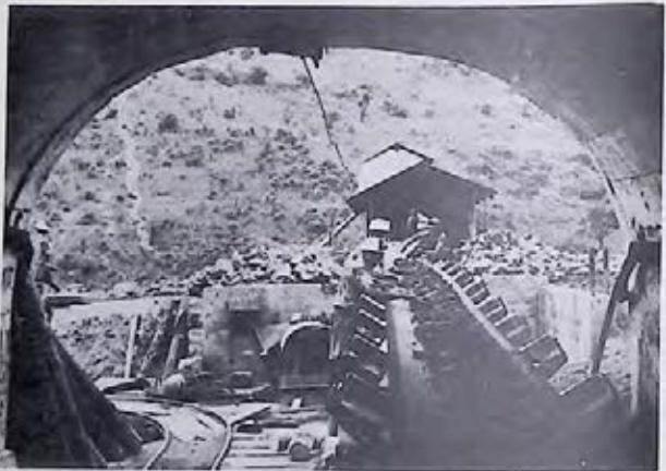
Fig. 111. This dramatic photograph shows the exit of the Okpara mine with a close-up of the conveyor belt. In the background you can see a miners' footpath. Several footpaths lead over the hills to the Okpara mine, since a large proportion of the miners come not from Enugu township but from neighbouring villages such as Nsude and Enugu Ngwo.
