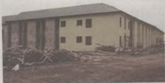
School of Nursing Students' Hostel complex Lafia, under construction
