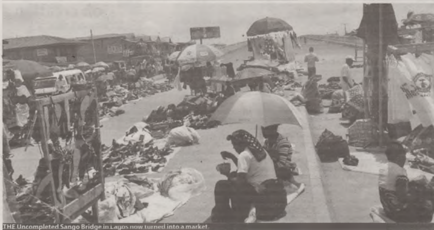
THE Uncompleted Sango Bridge in Lagos now turned into a market.
