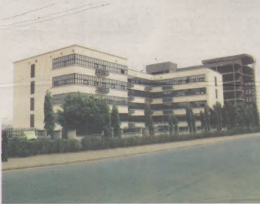
THE Federal Ministry of Education, Annex, Central Area, Abuja
