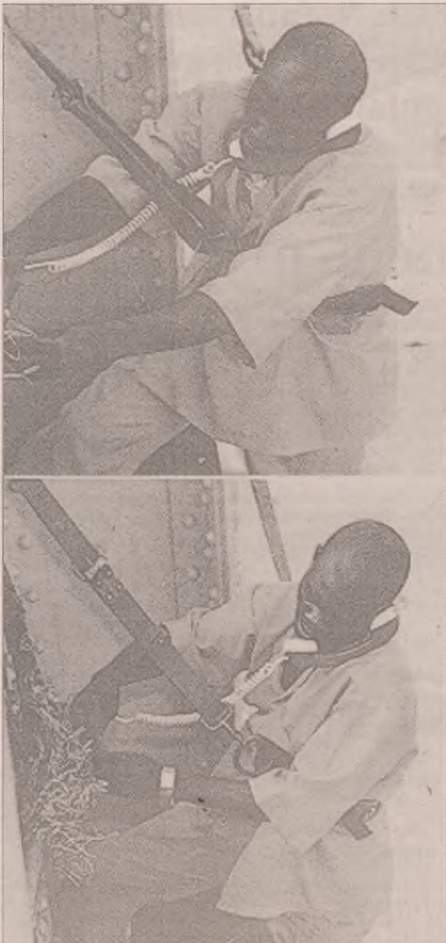
Dignity in labour: Abdullahi Idris (top) and Stephen Goja, (below), undertake repair work on NITEL cables over the River Benue; they took enormous risks by suspending themselves over the river to repair faults in the joints of a primary cable measuring about 165 metres which had
