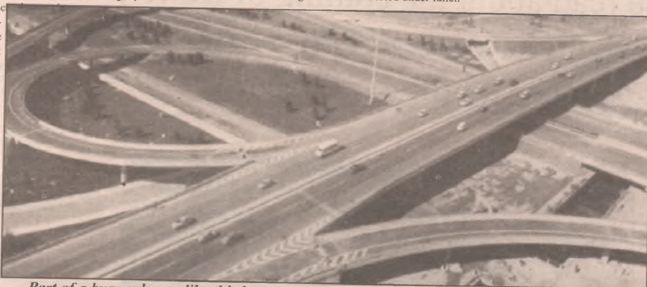
Part of a busy sub-way like this is now a collection of rubble and waste after the earthquake
