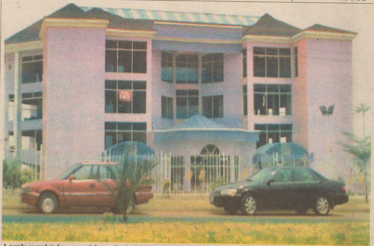
A newly completed commercial complex in Jabi district, Abuja
