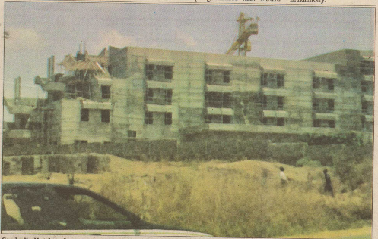
Sandralia Hotel, under construction in Utako district, Abuja
