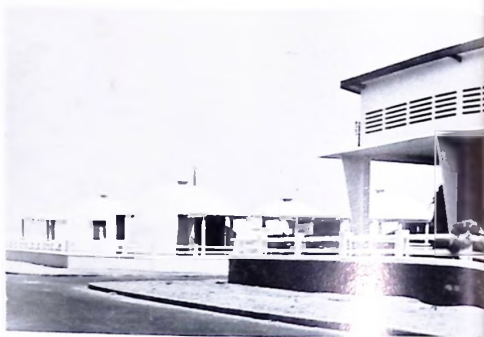
47. Ultra-modern housing at Fann. The houses on the left are made up of circular rooms built by pouring the setting cement over a balloon frame. The projection on the conventional house is to increase ventilation.
