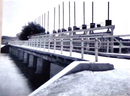
40. The Barrage on the Taouey tributary of the Senegal River. When the Senegal floods, its waters surge up this tributary and the sluice gates are opened—generally from mid-July to mid-November. Thereafter they are closed to prevent the inlet of brackish tidal water.
