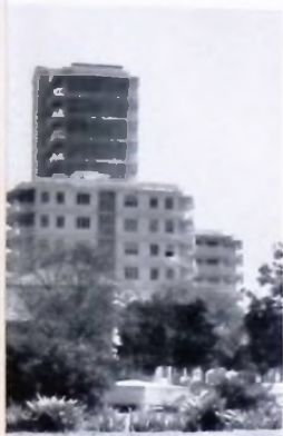
46. Thirteen storey block of apartments
