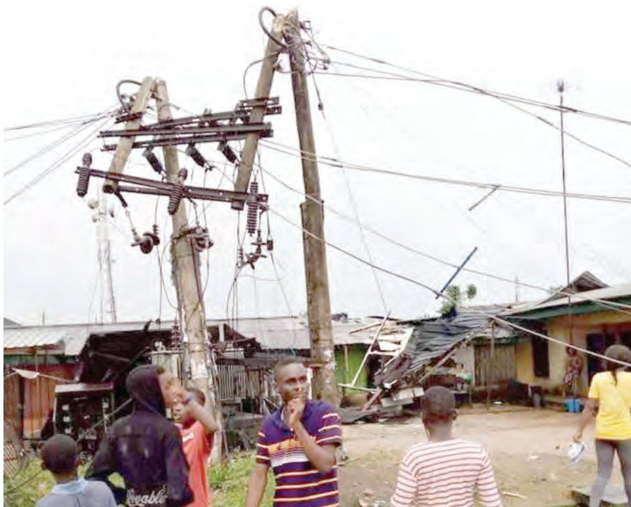
■ Damaged houses and electric poles in Oyigbo community in Rivers State after a heavy rainfall
