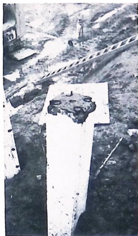
The lower element is driven.
