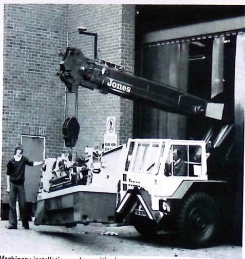
Machinery installation and repositioning
