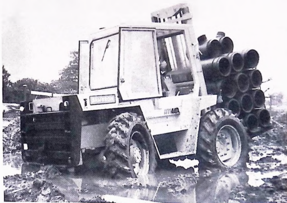
Diesel trucks are still used exclusively for rough terrain work.
