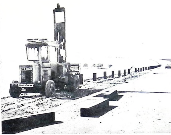
The mobile hydraulic hammer can be used for cutting trenches, driving posts, compacting fill, punching holes and even cutting recesses in asphalt roads for reflector-studs or cats' eyes.
