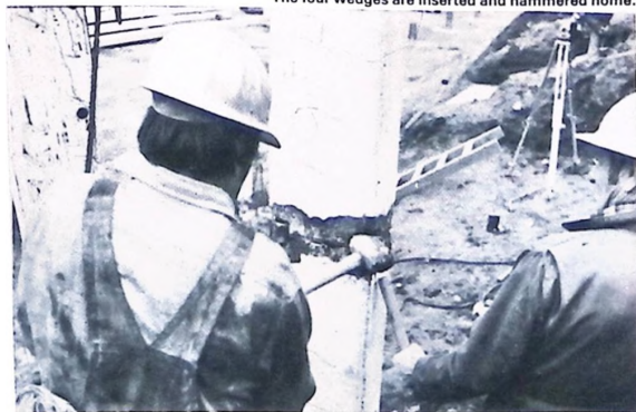
The four wedges are inserted and hammered home.
