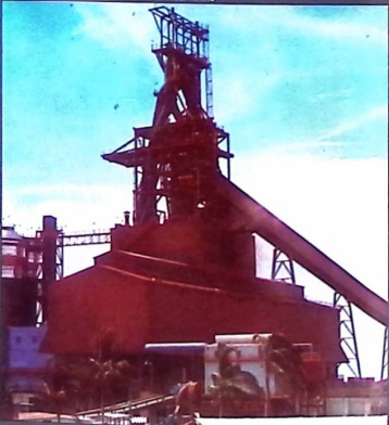
STAHLWERKE PEINE SALZGITTER A.G., Salzgitter, WEST GERMANY Pusher-type 300 t/h capacity each, slab reheating furnaces to feed a 90" hot strip mill
