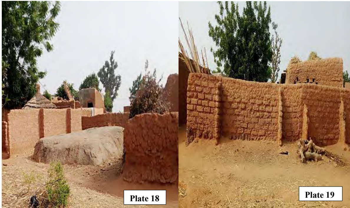
Plates 18 and 19: Typical compounds at the rusty Durbi Takusheyi settlement
