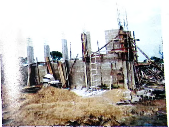
1000-seat Large Lecture Theatre for College of Engineering under construction
