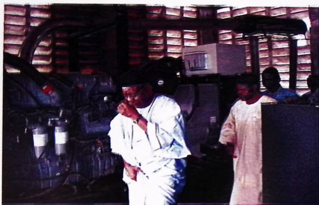
Commissioning of a New 500 KVA Generator
