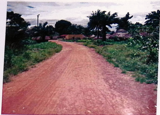
Rural Access Road constructed by author
