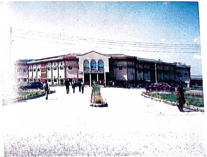
Completed College of Food Technology Building
