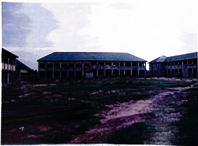
Construction of lecture Hall Block for College of Agronomy
