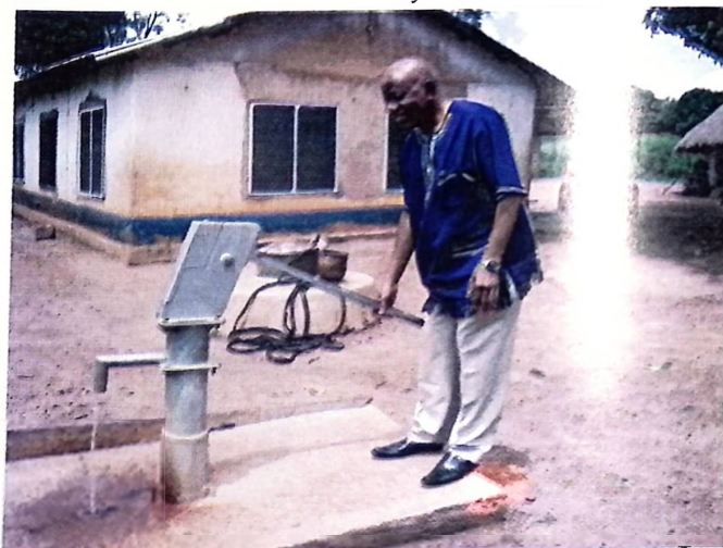
Borehole at NKST Primary School, Iyon, a donation by author
