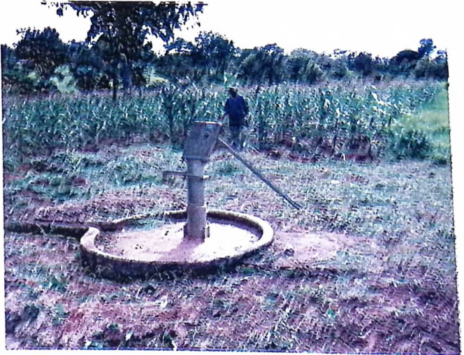
Borehole at Uza village
