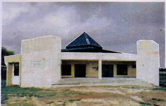
A newly completed large lecture theatre for College of Engineering
