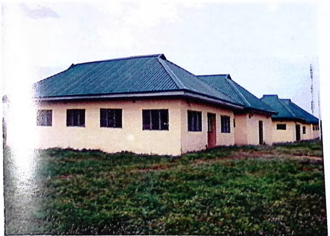
Newly completed Veterinary Teaching Hospital, UAM
