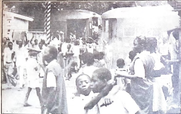
Yaba railway crossing blocked by overturned Coaches
