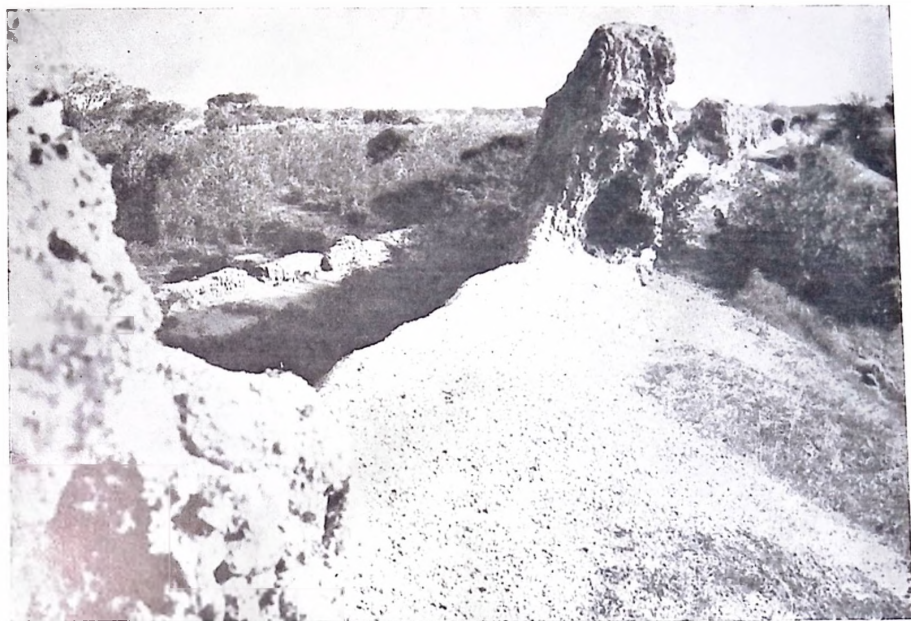
Section of Wall near Kofar Duka Wuyal showing small wall on outer edge of moat
