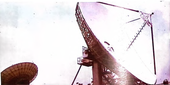
Digital Satellite Earth Station, Victoria Island, Lagos
