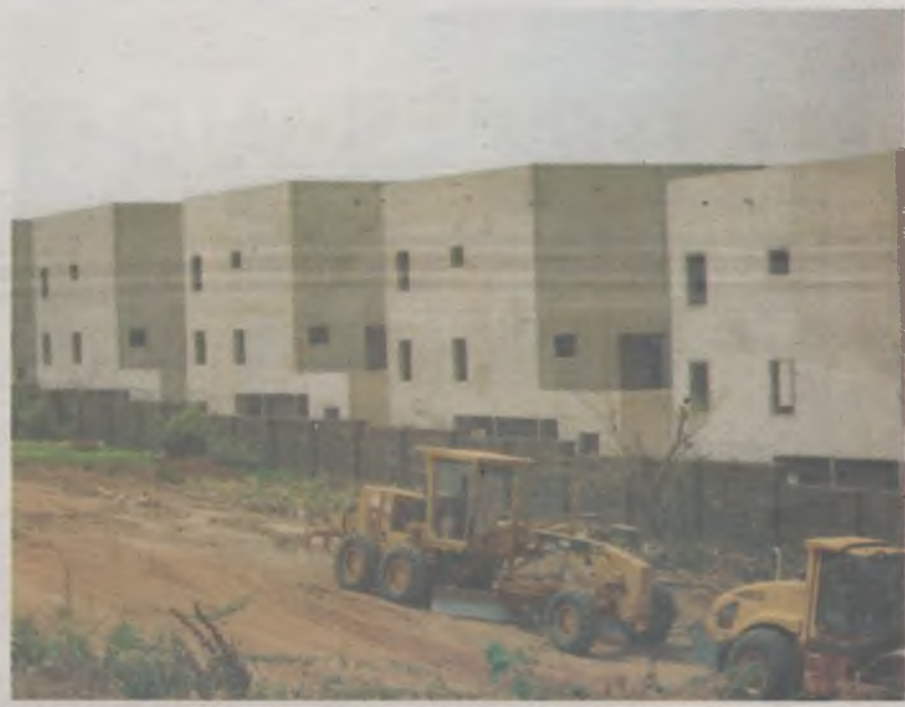
BLOCK of apartments nearing completion in Maitama, Abuja
