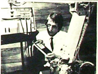
The portable "Placements" robot from Britain, highly versatile capability as a permanent fixture or as a mobile back-up for a range of work, including spraying, quality control, tinning and assembly.
