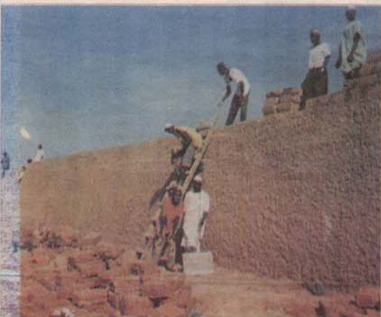
Reconstruction of Kano walls in progress
