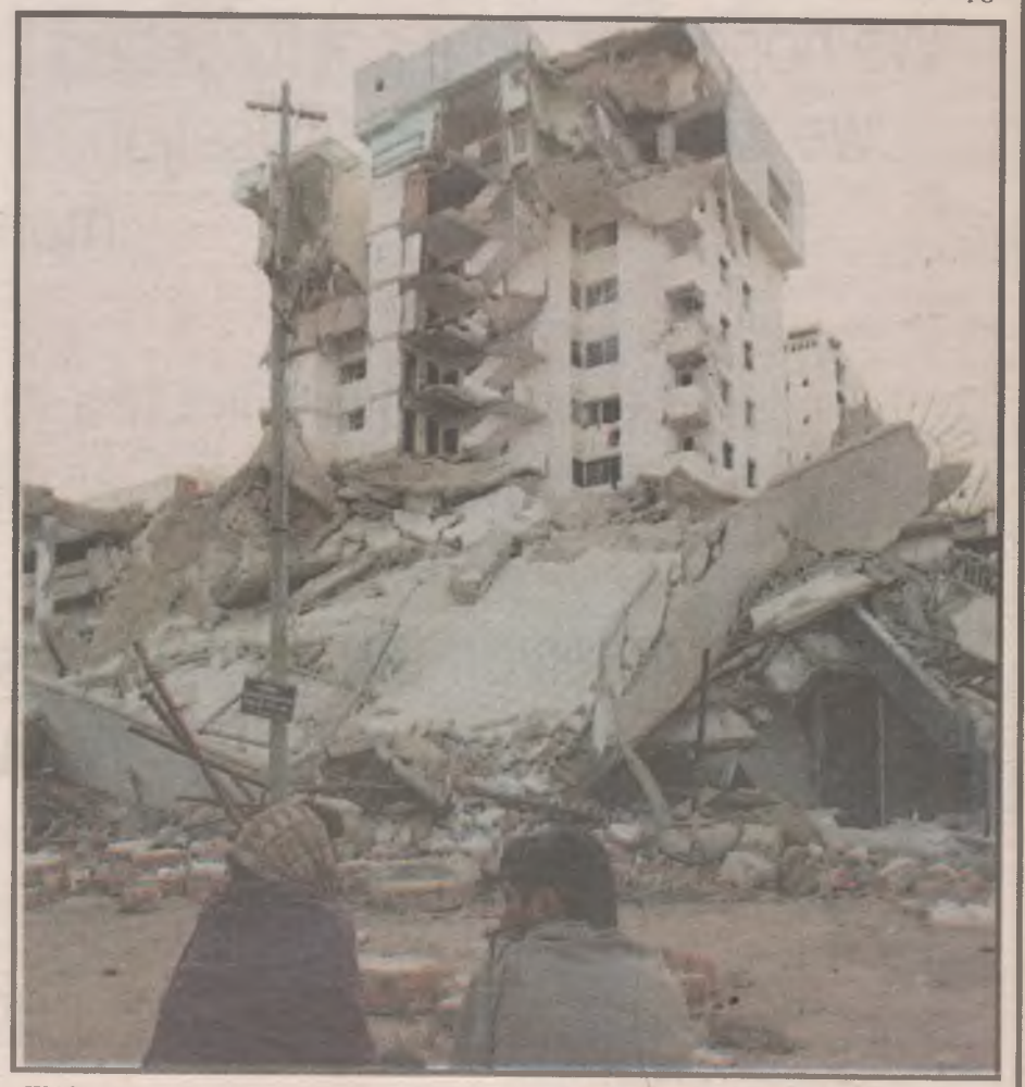
Workers take a break as they wait for a crane to arrive to help move large slabs of concrete in Ahmedabad, January 27, 2001. Several residents are still trapped under the debris. More than 15,000 people were feared dead as the worst earthquake to hit India in 50 years, measuring 6.9 on the Richter scale, shook the entire western state of Gujarat. Pix: AFP
