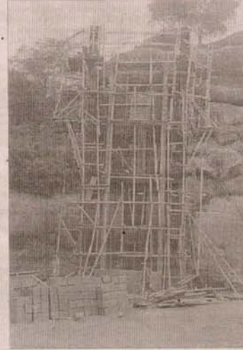
The glass elevator nearing completion at Olumo Rock Ogun State.
