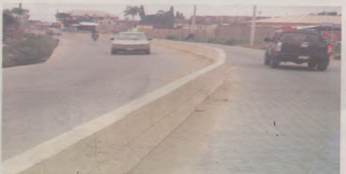
SIBIRI-Imude Road in Ijanikin under construction by the Lagos State Government
