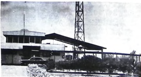
VON transmitting station at Ikorodu showing one of the many masts which will carry your message over thousands of kilometres to your loved ones abroad.
