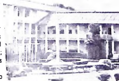
The front view of F.R.C.N. Lagos building at Ikoyi, Lagos
